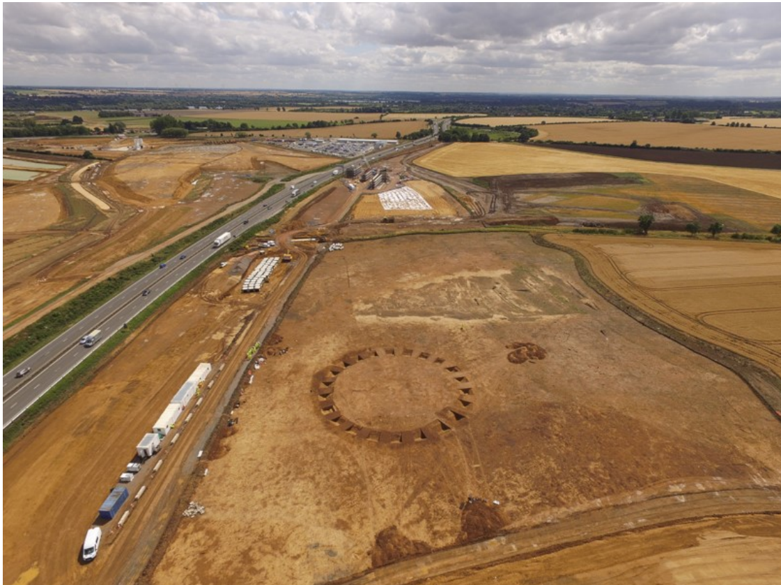
Fig 1 – A small section of the A14 under construction (© MOLA Headland Infrastructure)
