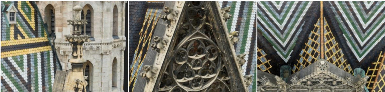
Fig. 3. High-resolution, photorealistic renderings of the textured 3D-model. Areas without TLS points (see Fig. 1) could be modelled completely.
