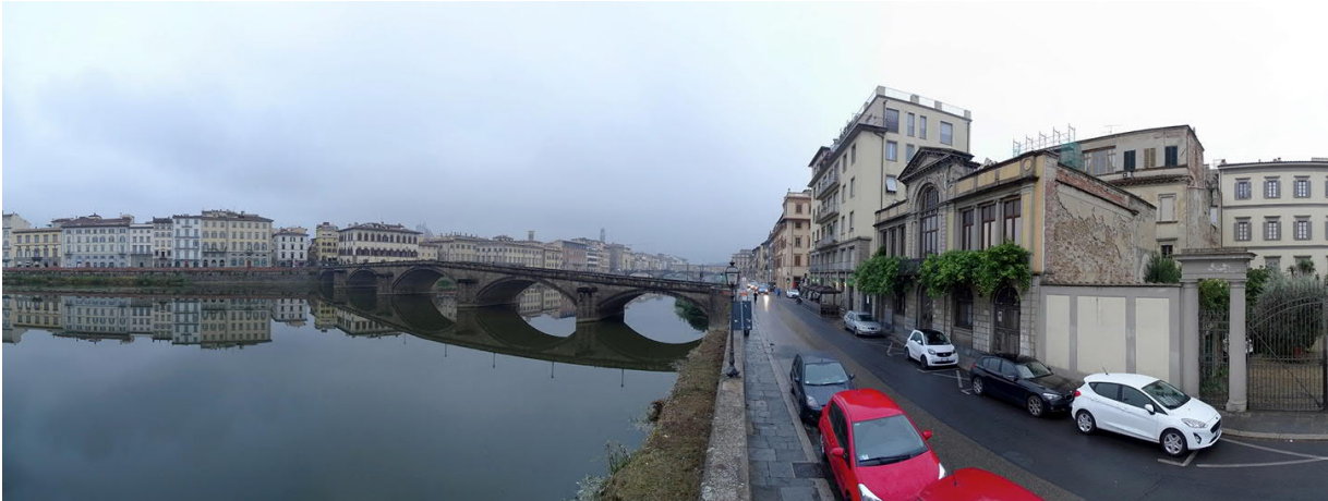
Fig.1. Main front of the Galleria Bellini, toward Arno River
