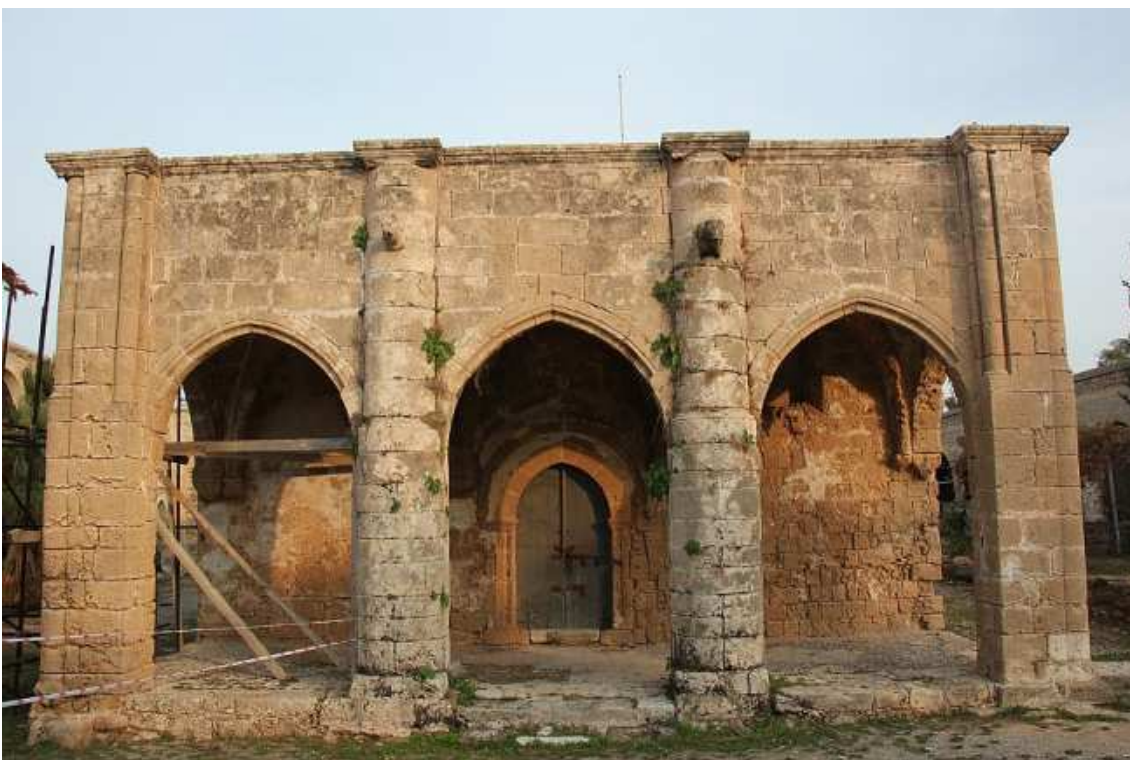
Fig. 2 – Front of the katholikon (Copyright: Carmine Canaletti, February 2015)
