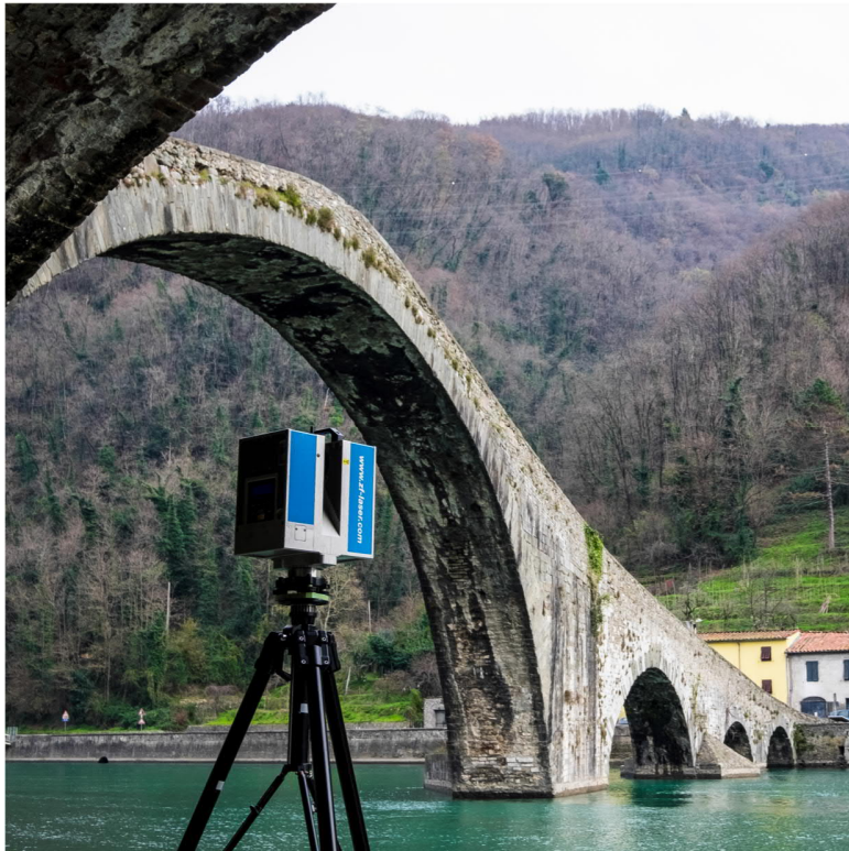
Fig. 1. One of the 44 laser scanner stations in Maddalena's Bridge
