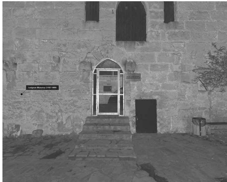
Fig. 13. Insertion of masonry survey into the point cloud - Lusignan Masonry (1192-1489)
