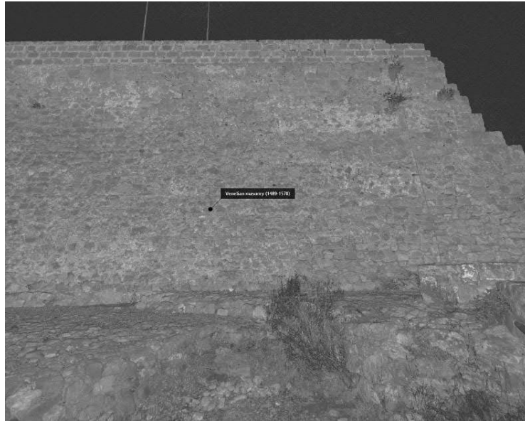
Fig. 16. Insertion of masonry survey into the point cloud - Venetian Masonry (1489-1570)
