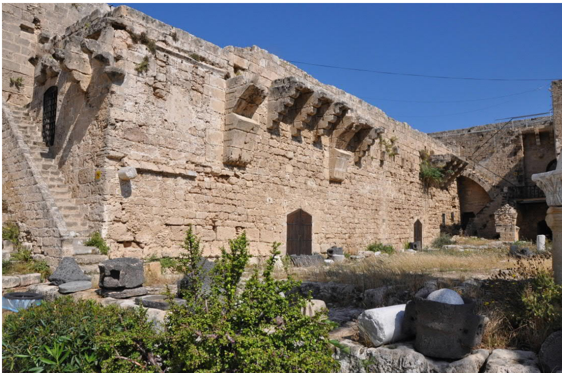
Fig. 4. Masonry analysis: balcony shelves on Lusignan masonry testify the past presence of upper storeys (© E. Valletta)
