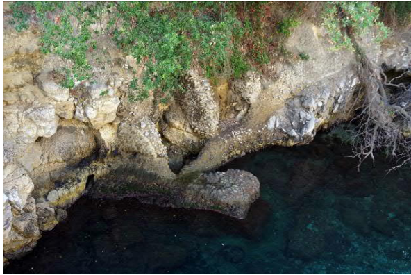
Fig. 10. Pier in front of the niche façade in the inner harbour (© M. Reinfeld)
