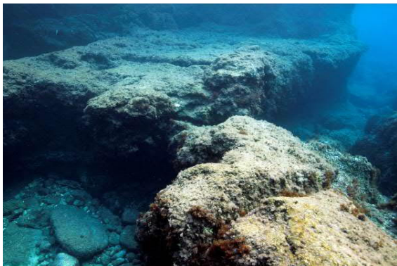
Fig. 19. Cuttings in the bedrock of the harbour basin attesting the use of scaffoldings for caissons into which the caementitium foundation of the mole had been set (© M. Reinfeld)
